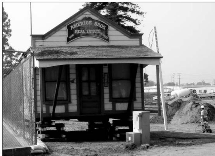
*2011: The Amerige Brother's Real Estate Office is temporarily positioned awaiting being placed on its new foundation.*
